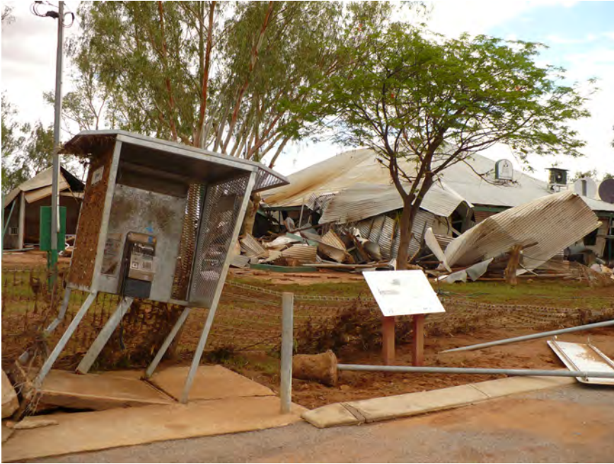
Figure 2b Flood damage at Gascoyne Junction townsite (December 2010). Photograph: J Stretch
