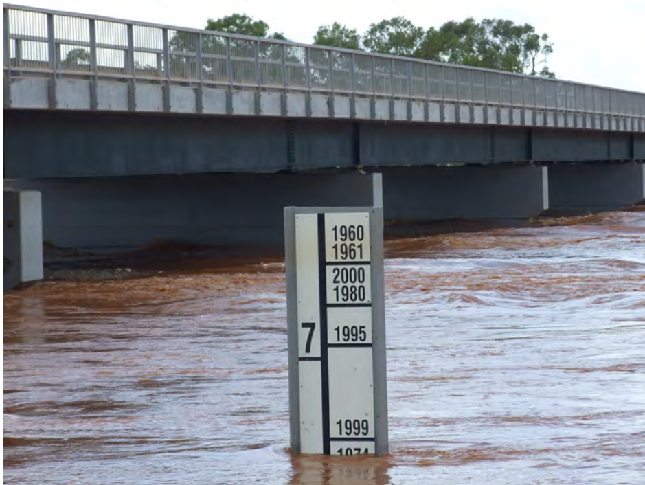
Figure 10 Gascoyne River flood waters at Nine Mile Bridge, near Carnarvon
