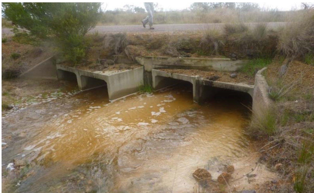
Plate 14 Neridup Creek flowing through box culverts under Fisheries Road (taken 29/07/2009)
