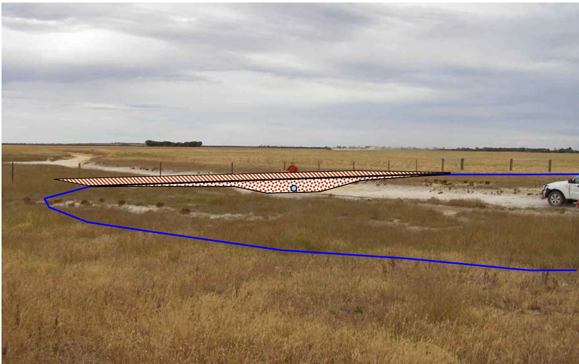
Figure 14 Possible detention area for controlling water flow. The hatched area represents the wall constructed across the drain with a pipe in the base; the blue line represents the extent of water detained behind the wall when full.
