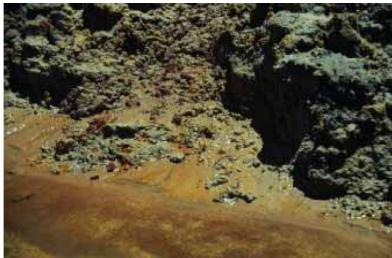
Photo 2: One of the few major seepage zones. Note: the collapse of material at the seepage zone which is in the centre of the photograph.
