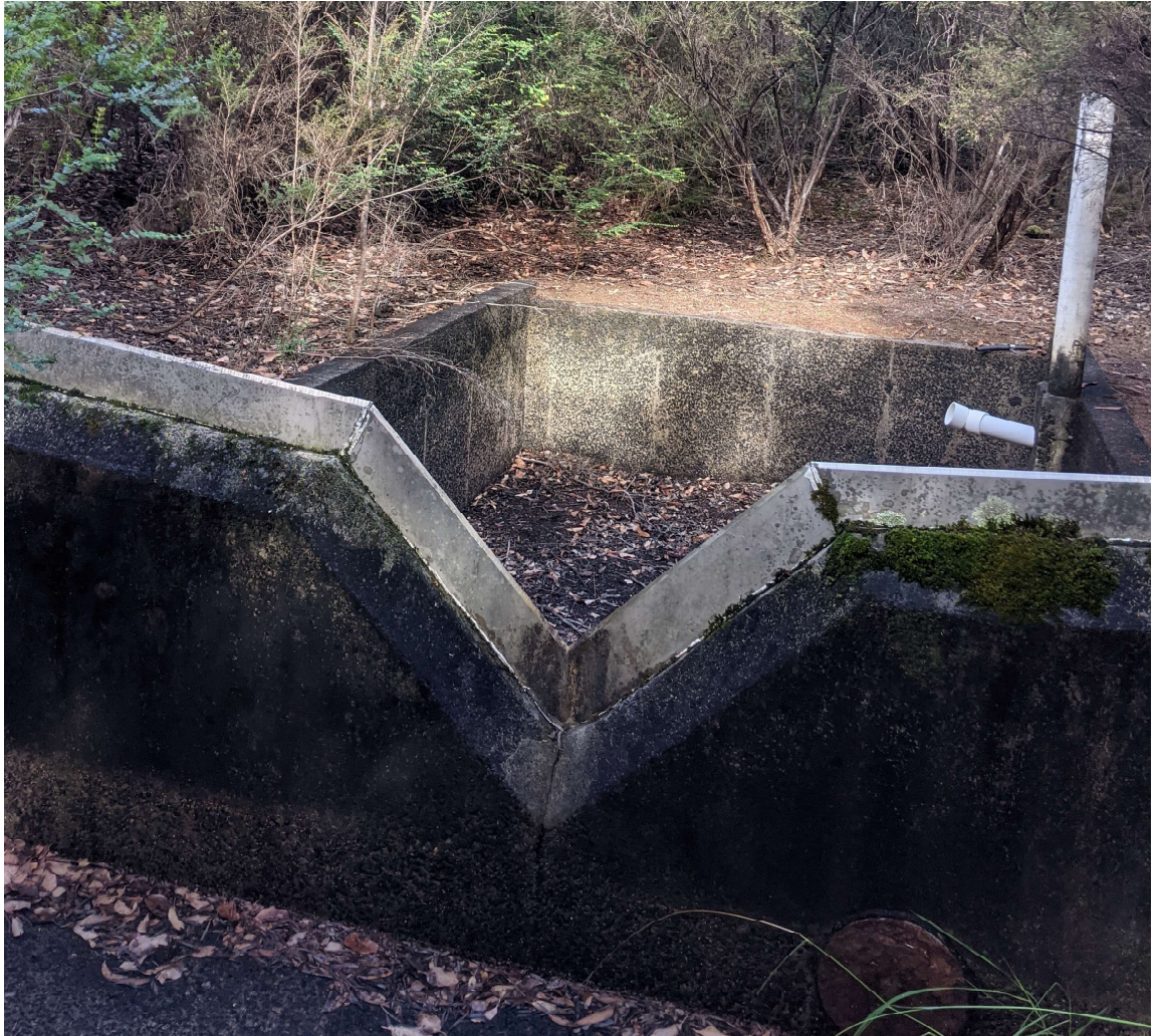
Figure 4.1: Lewin North stream gauging weir, looking upstream
