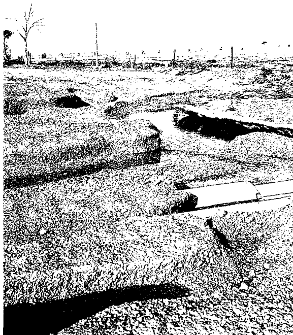
13. Damage to a flood way following one intense rainfall event.
