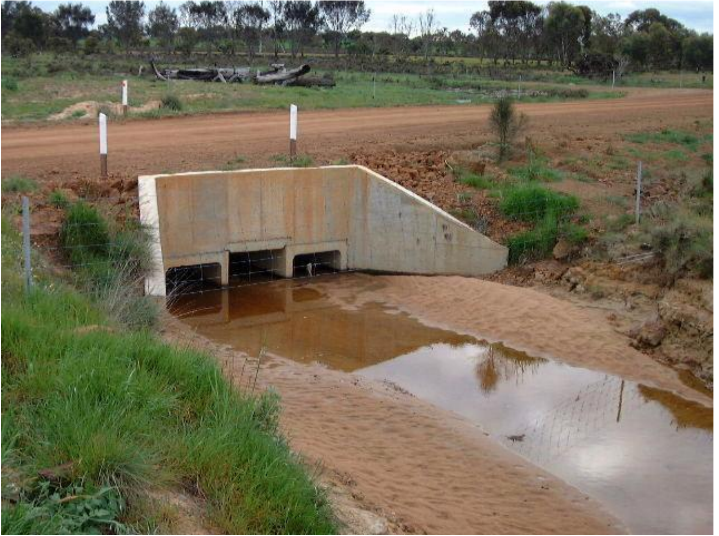
Image 3: Soil loss by water erosion can block drainage culverts, cause roadway flooding and, in some places, cause further streambank erosion.
