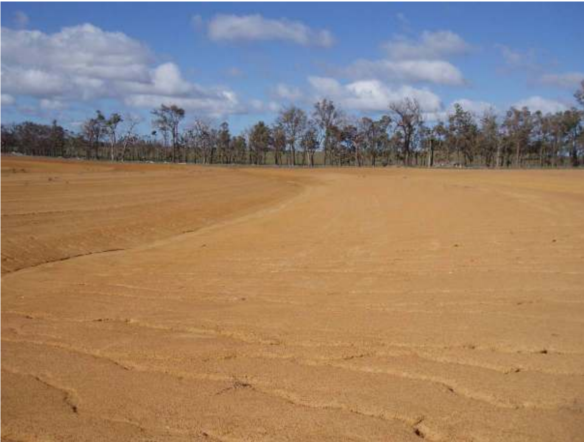
Figure 8 Roaded catchment to improve collection of rainfall run-off in Great Southern, Western Australia (Stanton 2005)
